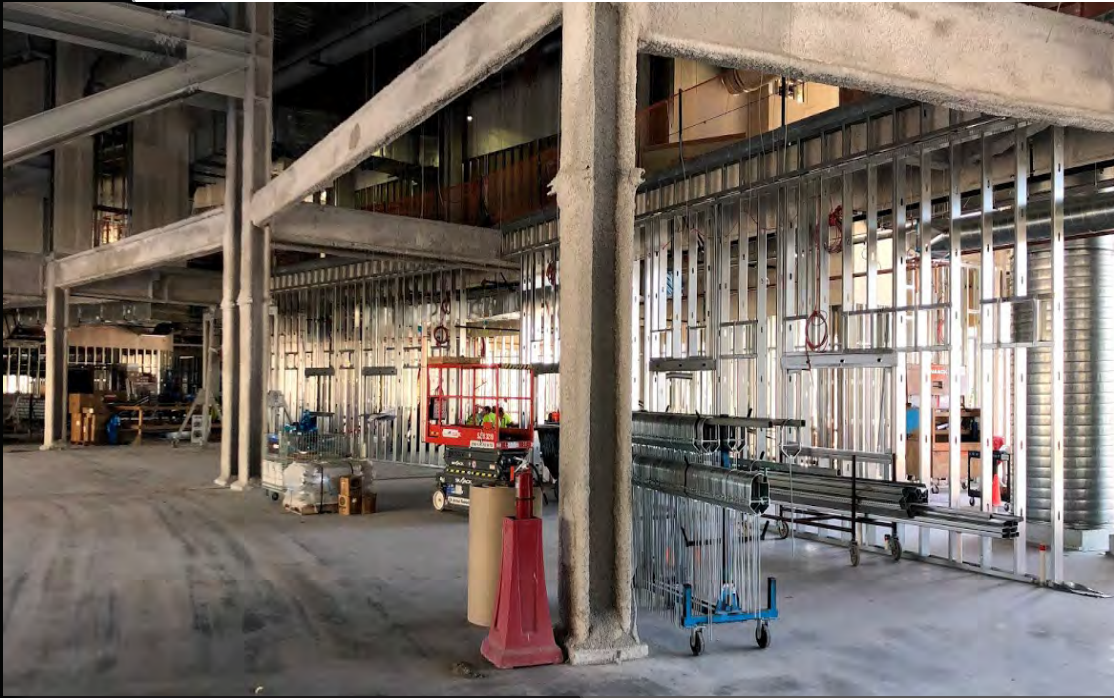
Above: Main Concourse metal stud framing. Below: Enclos laydown area.
